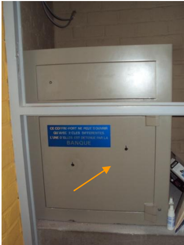
Photo 1 Coffre-fort couloir direction
