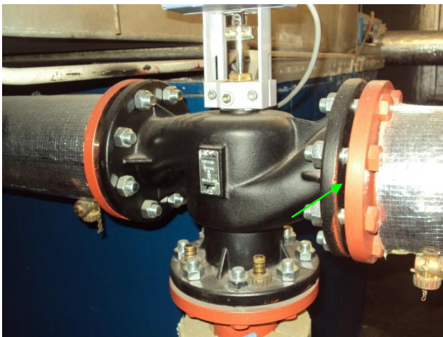
Photo 3 Joint de bride chaufferie
