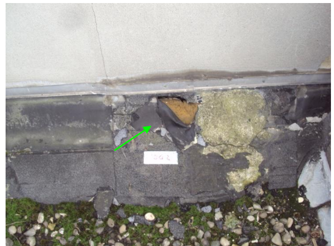
Photo 4 Roofing toit couloir
