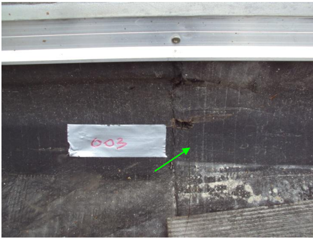
Photo 5 Roofing toit couloir
